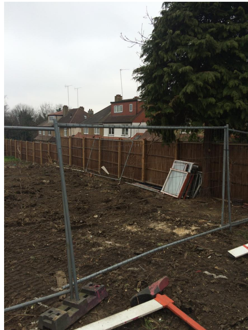
Site looking at rear of Albert Road properties
